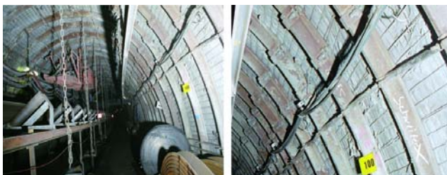
Figure 1: Yielding roadway arch support with concrete material backfilling
